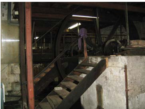
Installations de transmission
